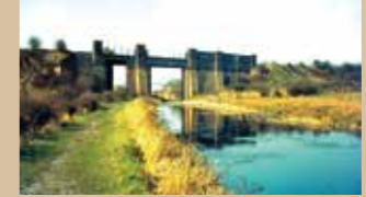
The former Great Northern Railway bridge over the Nottingham Canal. Photo courtesy of Michael Golds
